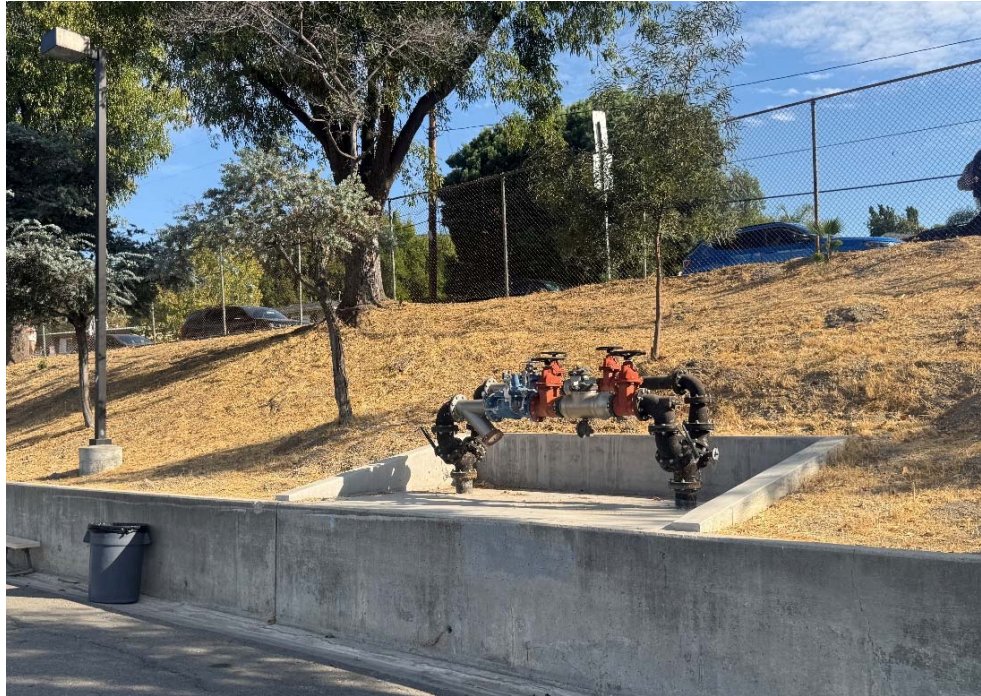
Figure 29. Taft HS – Backflow Prevention System at Santa Rita Street (OIG Photo– October 4, 2024)
