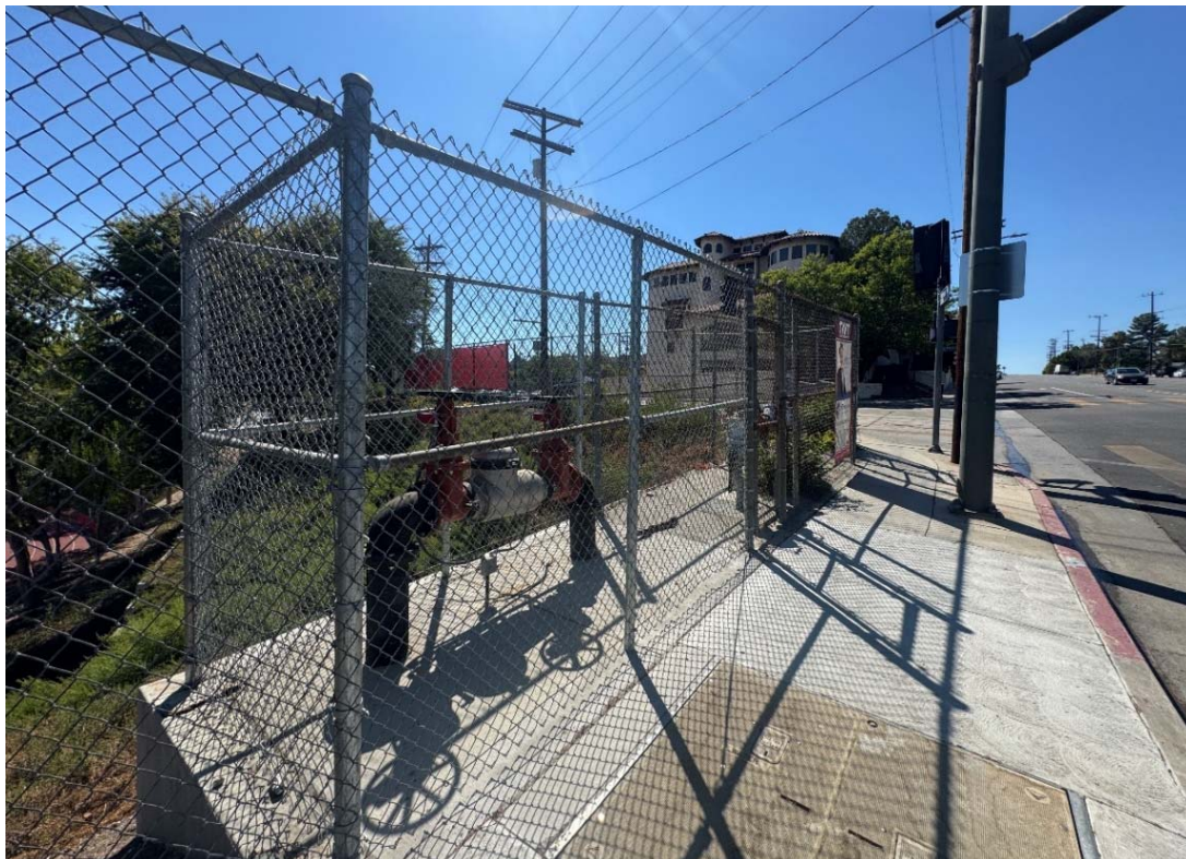
Figure 35. Taft HS – Backflow Prevention System at Campus Northwest Corner (OIG Photo– October 4, 2024)
